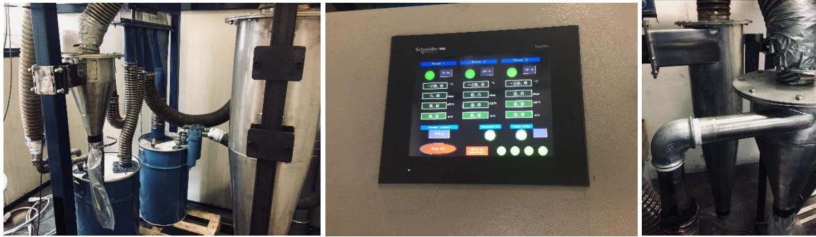
Figure 3 From the left: the cyclones and collecting drums, the PLC running the project, detail of the installed cyclones
